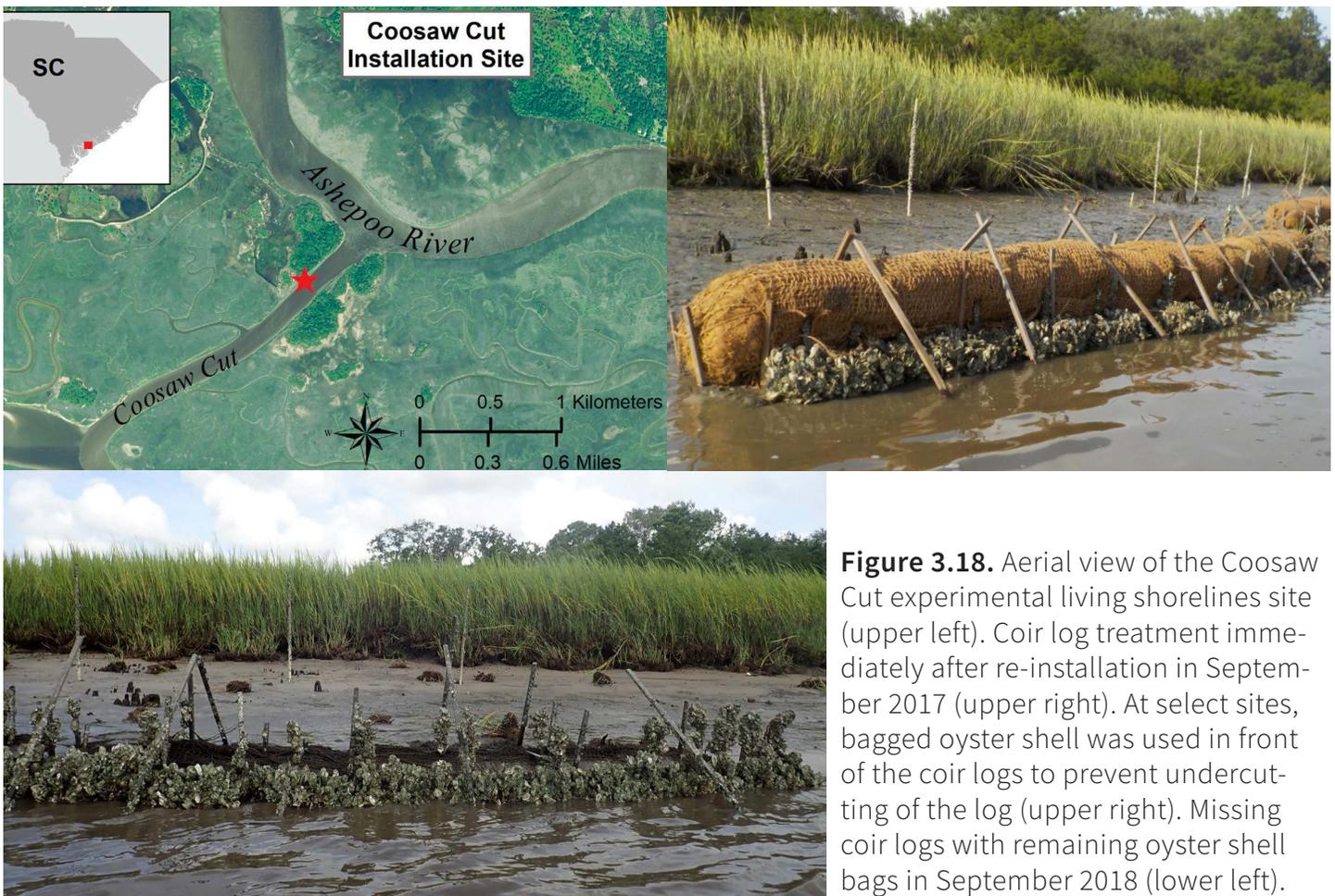
**Figure 3.18.** Aerial view of the Coosaw Cut experimental living shorelines site (upper left). Coir log treatment immediately after re-installation in September 2017 (upper right). At select sites, bagged oyster shell was used in front of the coir logs to prevent undercutting of the log (upper right). Missing coir logs with remaining oyster shell bags in September 2018 (lower left).
