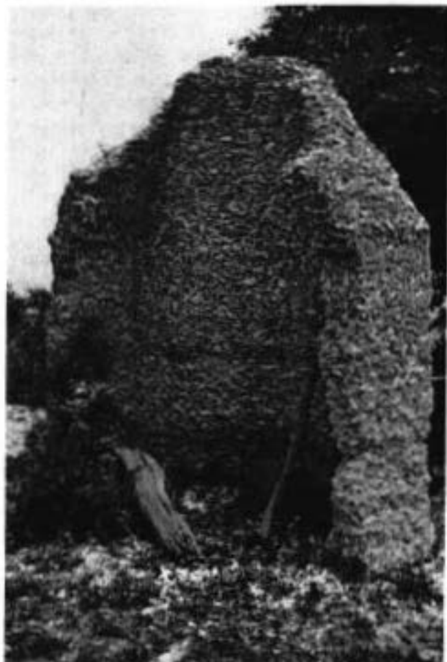
FIGURE 13—A portion of the tabby ruins located at Hague Point on Daufuskie Island.
