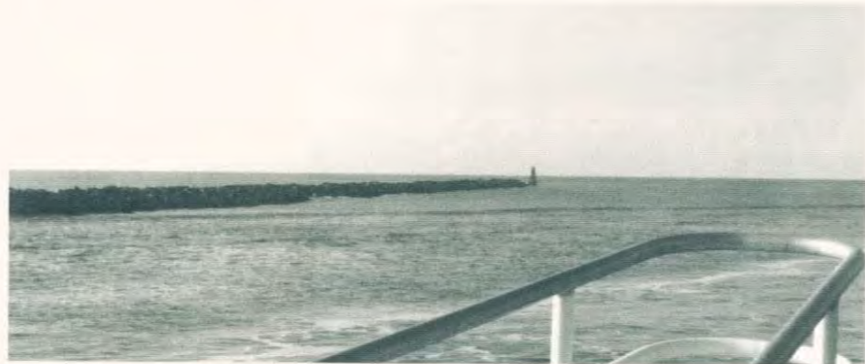
The Little River jetties completed in 1983 by the U.S. Army Corps of Engineers. This allowed deep draft vessels to transit the bar on any tide. (photo from the author)
