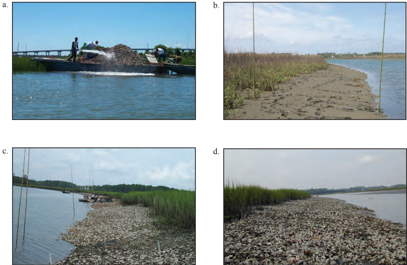
Figure 1. Large-scale restoration activities: a - planting shell with barge and water cannon; b - shoreline prior to planting; c - shoreline immediately after planting; d - shoreline with newly planted area
